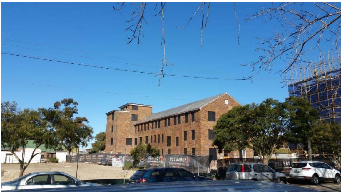
Figure 5: Former South Sydney Hospital site: former Administration building for water re-use and pedestrian connection to aquatic centre and playing fields along fabric hoarding line
